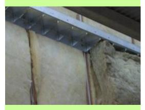
After removing the panels and old insulation of the gable walls, 2 layers of insulation were added.
