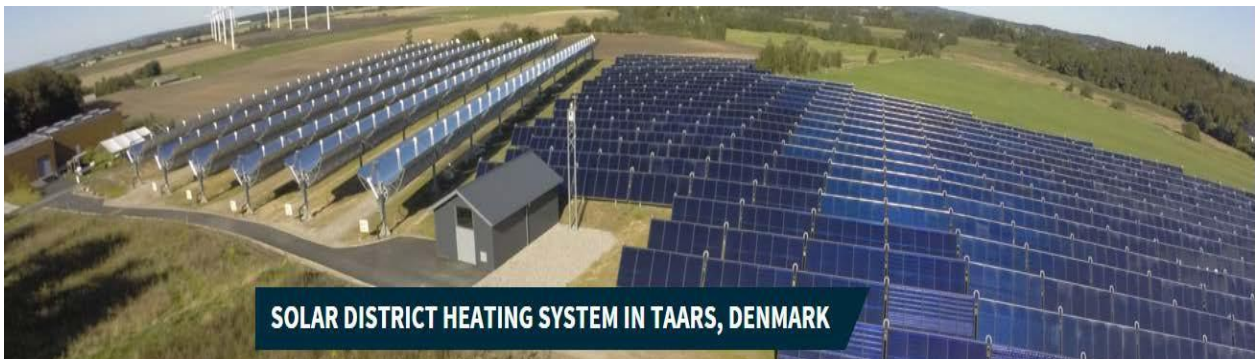
Fig. 2 The hybrid solar collector field of the Taars plant (Source: Aalborg CSP A/S).
