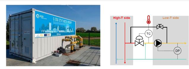
Figure 5. Supply-to-return mixing station: external view and simplified scheme (Source: [6])
