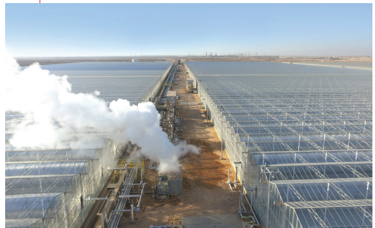
▲ The world's largest solar process heat plant Miraah in Oman was significantly enlarged in 2019 and now has an installed capacity of 300 MWth. Photo: GlassPoint Solar, Inc.
