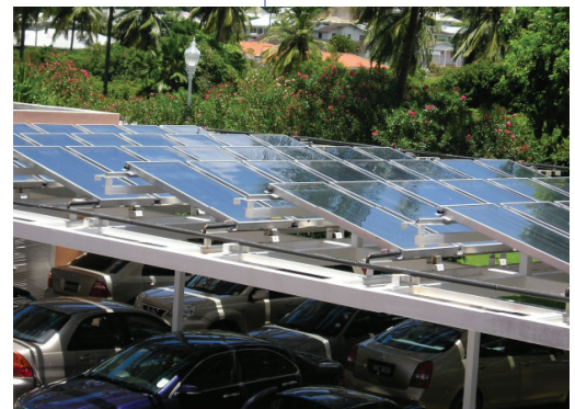
▲ 64 collectors on a carport supply the hot water for a resort in Barbados. Photo: Solar Dynamics
