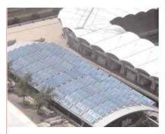
Solar district heating plant in the city of Graz with an installed capacity of I MWth (1400 m<sup>2</sup> collector area). (Source: S.O.L.I.D.)
