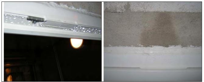
Figure 5.8: Condensation in the window frame, ventilation opening and wetting of the wall at the top side.
