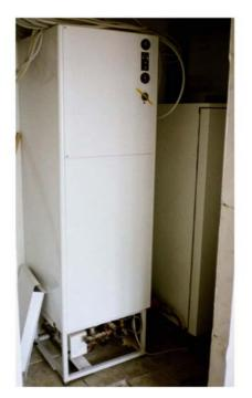
The system uses a standard solar domestic hot water tank with all components of the system integrated in the same cabinet as the tank. The dimensions of the cabinet are furthermore modular  $0.6 \times 0.6$  m, so that it easily fits into the utility room.
