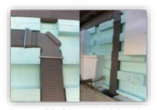
Figure 15 Façade insulations systems including air ducts
