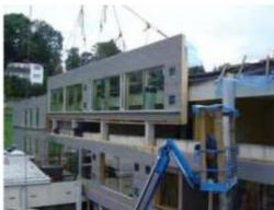
Figure 8 School in Schwanenstadt: installation of facade elements
