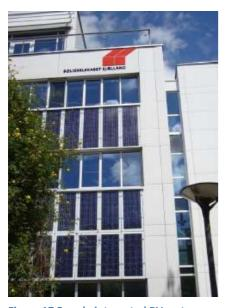
Figure 17 Façade integrated PV system, Office Building Roskilde
