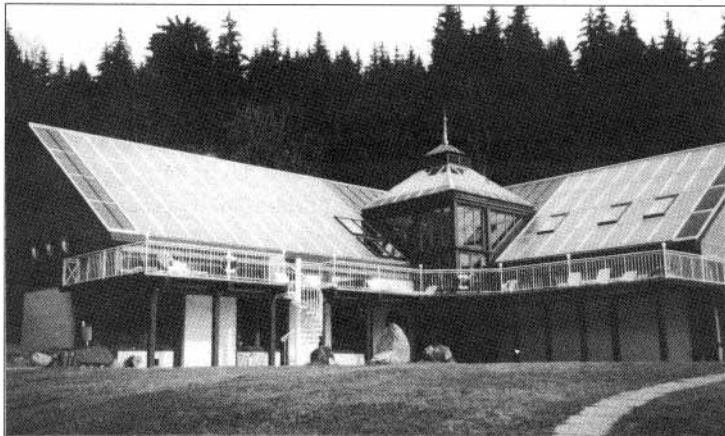
Solar installation in Austrian hotel.
